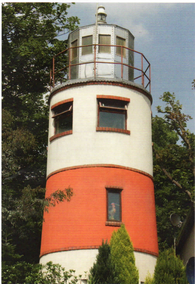
The Monton Lighthouse on the Bridgewater Canal near Eccles
